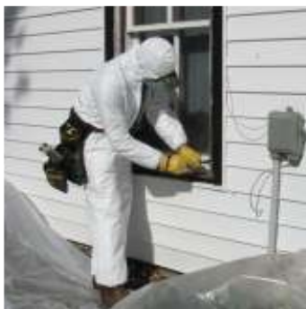
Weatherization crew performing window replacement
